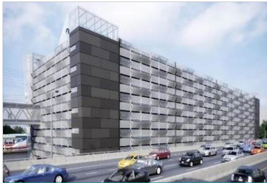
Stamford Station Parking Garage
