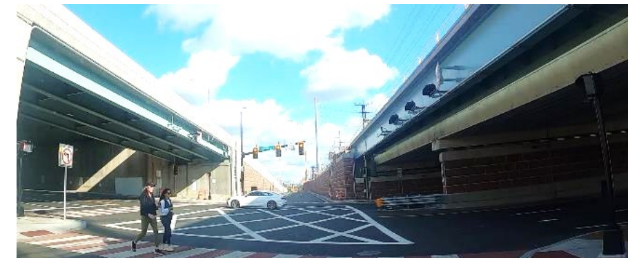
Critical North/South Arterials Connect I-95 to Downtown Stamford, South End, and other neighborhoods
