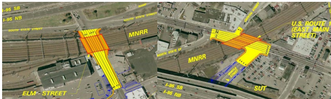
South Stamford Accessibility and MNRR Bridge Replacement SPN 135-301
